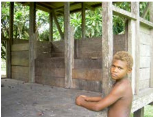
Figure 12.2 – Standard size fermentation boxes in a village fermentary, showing the heavy wood construction, the boxes raised off the ground and a roof protecting the boxes from rain
