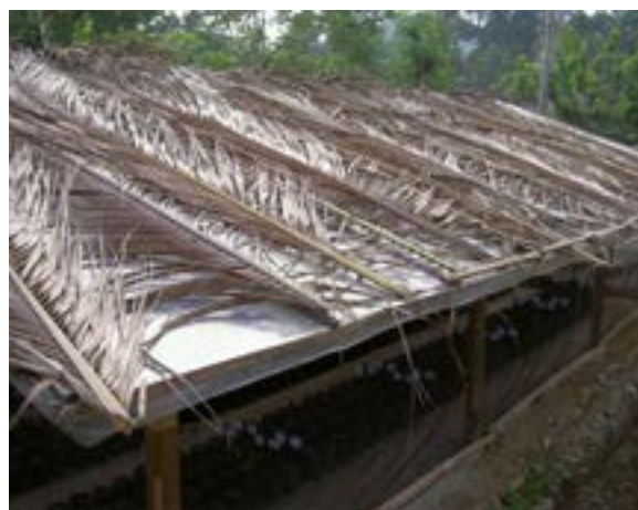
Figure 3.8 - Nursery roof with UV resistant plastic sheet covered with palm fronds for shade
