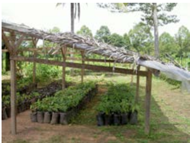
Figure 3.7 - Nursery construction – wood frame supporting a plastic cover and palm fronds; note the simple construction and overhang
