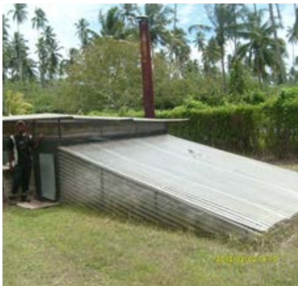
Figure 12.17 – Photos of combined solar/wood-fired kiln drier showing the polycarbonate sheets covering the black rock beds to guide hot air up through the drying rack that is protected by a polycarbonate roof that can be rolled off on rails to expose the beans; the wood-fired kiln can be lit during rain
